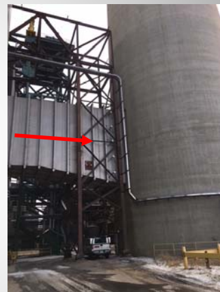
Exterior Stack Ports
